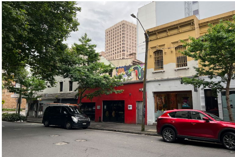
Figure 1-3: Reservoir Street frontage (Source: Curio Projects Oct 2022)
